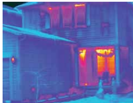
Homesol uses advanced building diagnostics tools including infrared thermal imaging.
